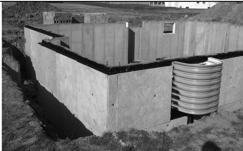
Figure R402.2.9(2) EXTERIOR BASEMENT INSULATION
