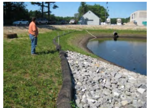
Continuous contained berms may be placed by hand, machinery or the sock may be filled on-site by a pneumatic blower.
