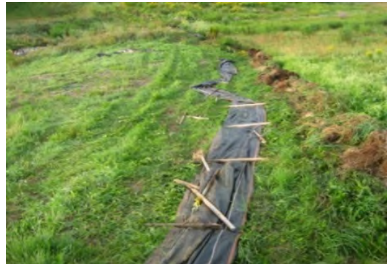
Sediment barriers should be removed when the area is stabilized. The collected sediments should be leveled, seeded and mulched.
