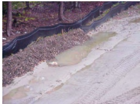
Damaged or otherwise ineffective sediment barriers should be replaced with new material or a different barrier measure.
