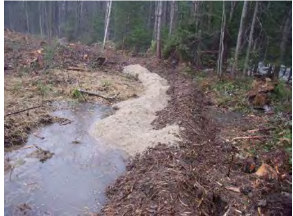
The spreader should be level and prevent channelization. In a temporary situation, erosion control mix or a berm of brush may provide the velocity reduction necessary to promote dispersion. Stone berms are recommended for larger flows.
