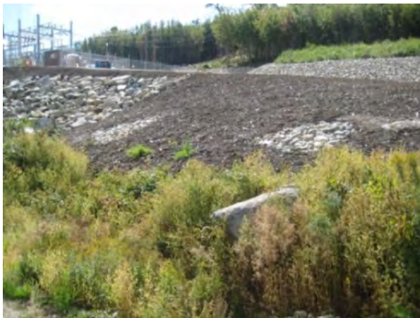
Groundwater drains, soil reinforcement or even a retaining wall may be necessary where the slope is failing due to groundwater seepage or soil instability.
