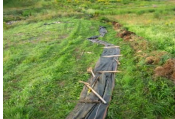
Sediment barriers should be removed when the area is stabilized. The collected sediments should be leveled, seeded and mulched.
