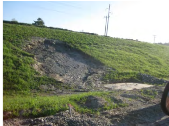
Slopes that will be revegetated should be no steeper than 2:1. Where the slope is to be mowed, the slope should be no steeper than 3:1 (4:1 is preferred for larger mowing equipment).
