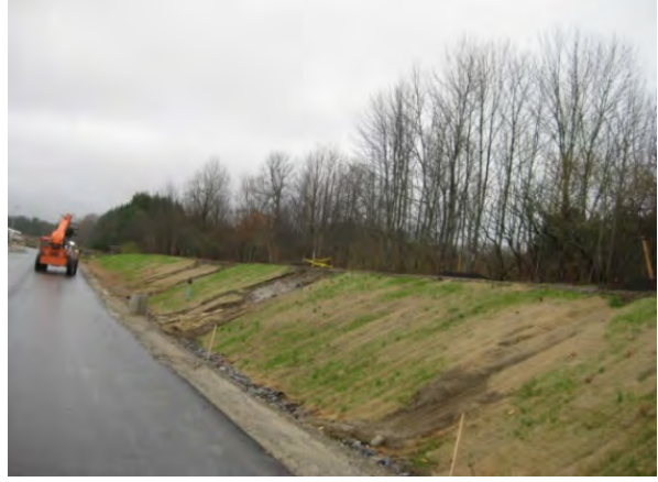
Slopes that will be revegetated should be no steeper than 2:1. Where the slope is to be mowed, the slope should be no steeper than 3:1 (4:1 is preferred for larger mowing equipment).
