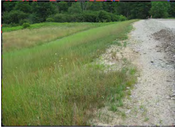
The entry angle from the channel to the level spreader should be no greater than 30 degrees to prevent scour and short circuiting.
